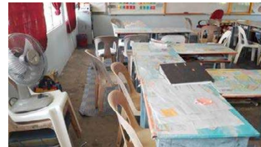
Figure 3: Unsuitable floor coverings
